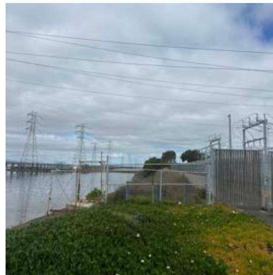
View D: PG&E Ravenswood Substation and transmission towers within Pond R2 from trail facing northwest.
