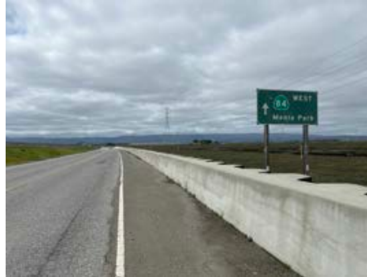
View D: Ravenswood frontage road north of SR 84 and south of Moseley Tract Marsh facing southwest.
