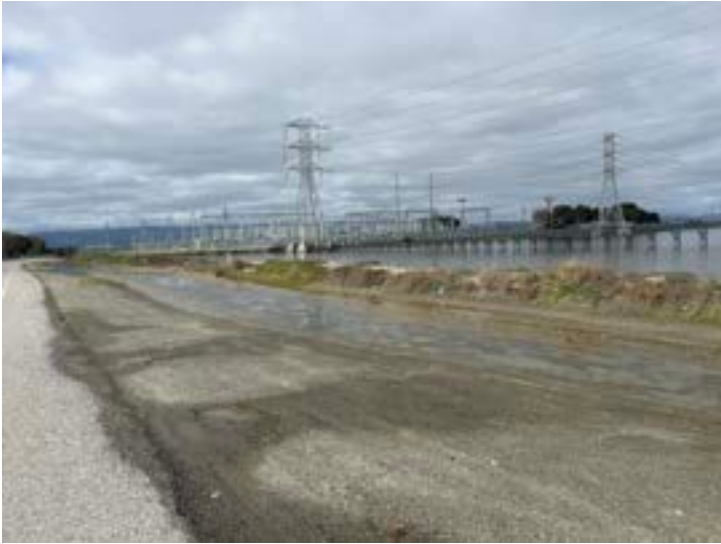
View A: Bay Trail facing west towards PG&E Ravenswood Substation.
