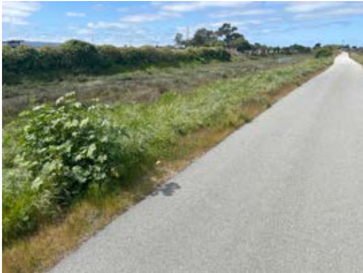
View A: Drainage channel east of Bay Trail facing northwest.
