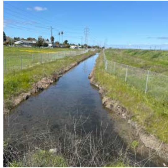
View B: Runnymede Drainage Ditch east of Martin Luther King Park facing north.
