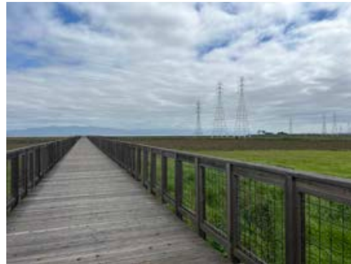
View D: Bay Trail Boardwalk north of Ravenwood Open Space Preserve facing east towards transmission towers and overhead power lines.
