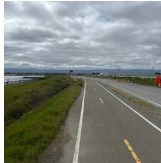
View B: Bay Trail and SR 84 north of Pond SF2 facing southwest.
