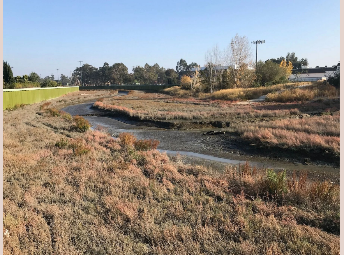
Reach 1 Project Area
