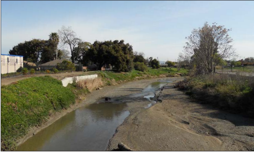
Viewpoint A: East Bayshore Road looking downstream (upper reach)
